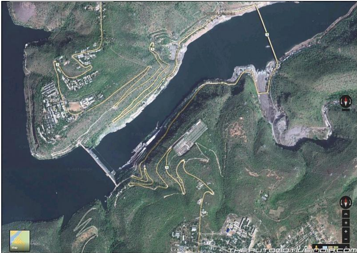
Fig-3: An Aerial View Of Srisailem Dam Site
